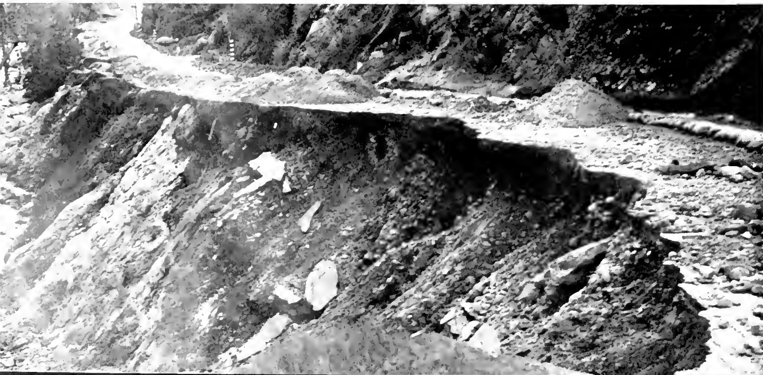
Flood waters rushing down Topanga Canyon to coast west of Santa Monica carried away huge sections of State Highway
